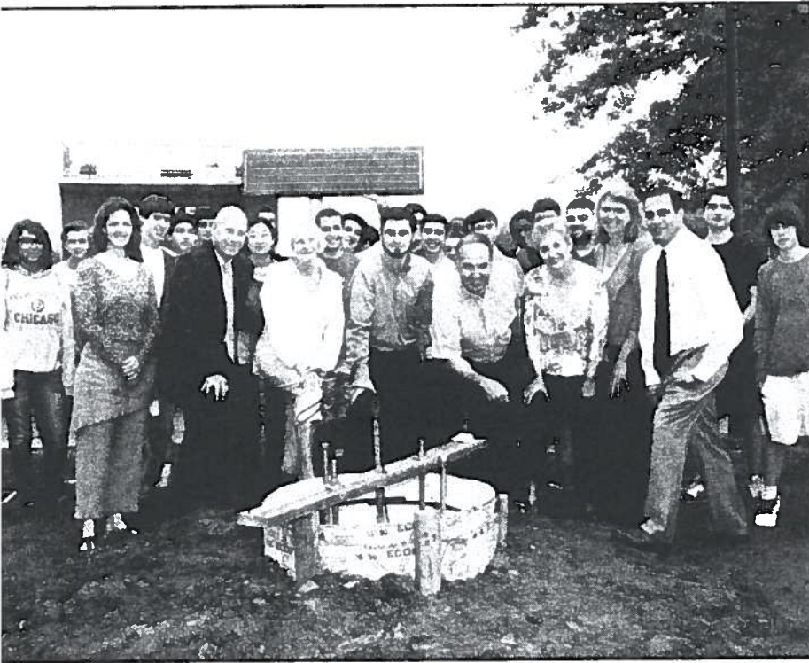
The gang's all here: foundation board members, teachers and students gather to check out the starting construction of Conard High School's new energy lab and display.
